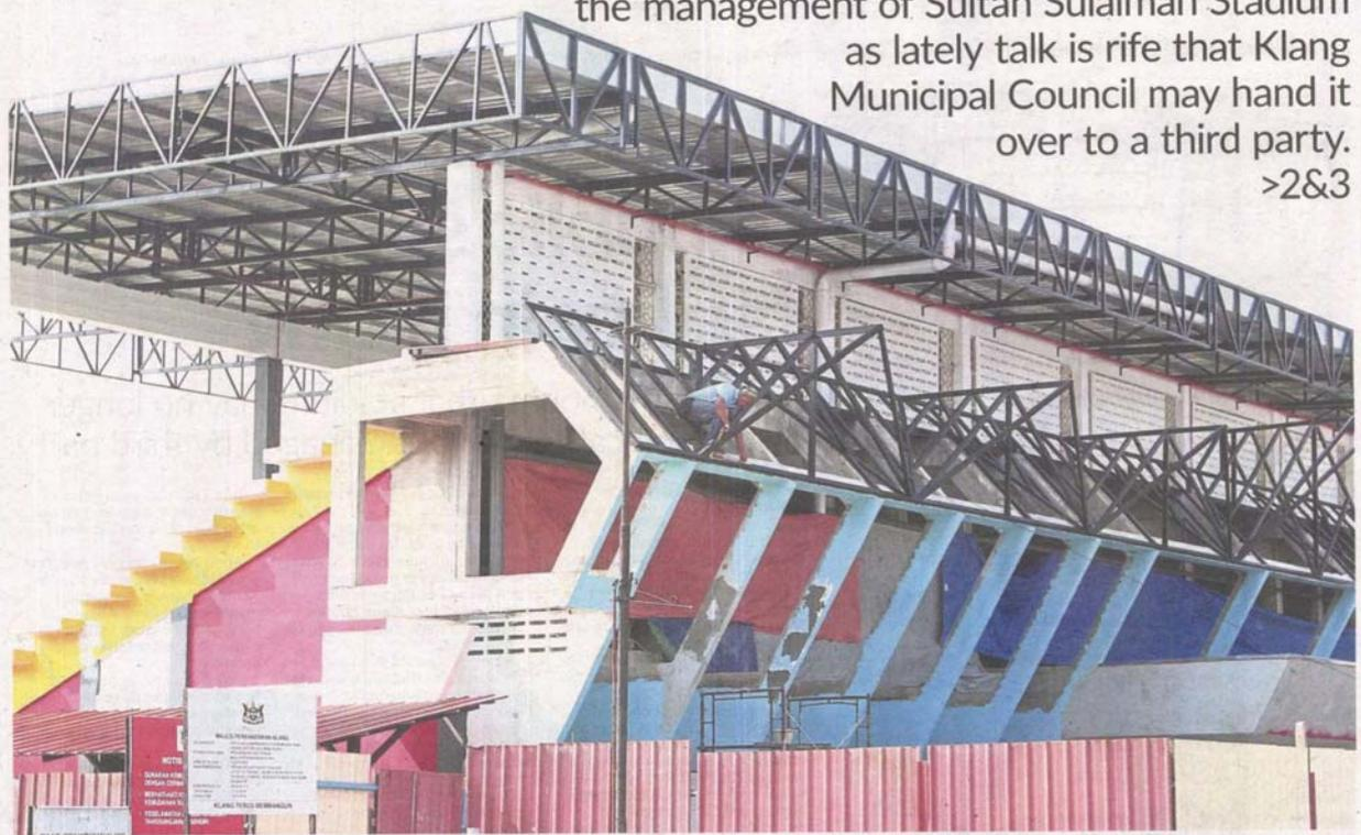
Fixing it: A worker painting the new metal frame of Sultan Sulaiman Stadium grandstand, which had to be replaced because of metal fatigue. — AZLINA ABDULLAH/The Star
